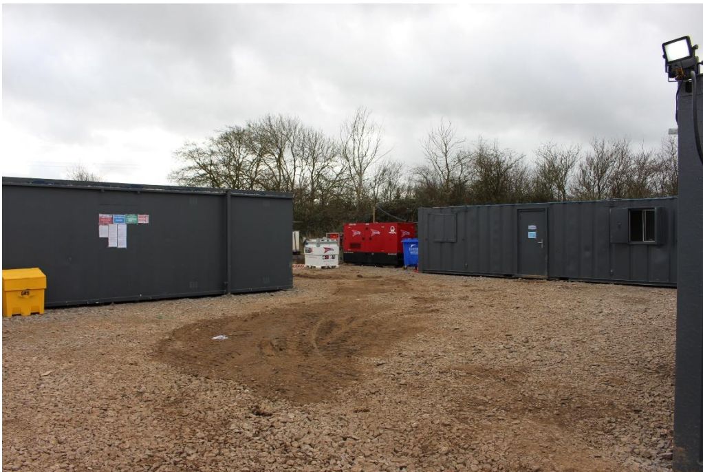
Plate 9: Establishment of the temporary construction compound(s)
