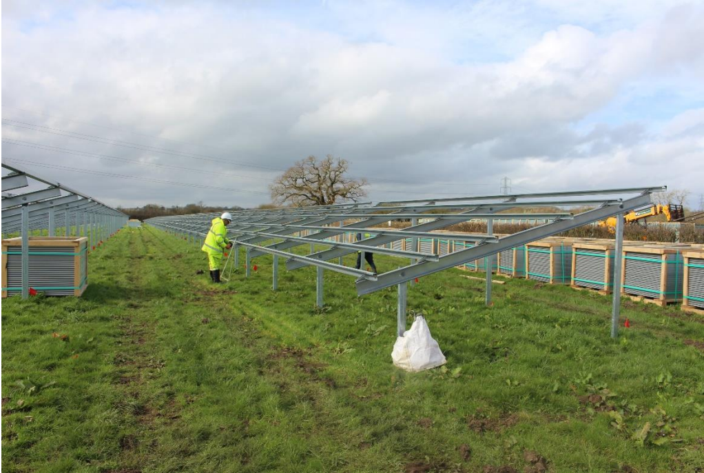
Plate 11d: Installation of Mounting Structures (4 of 4)
