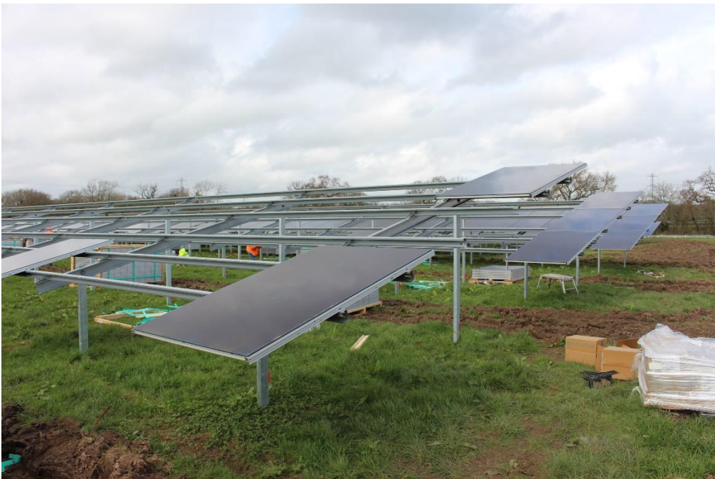
Plate 12: Mounting of PV Modules
