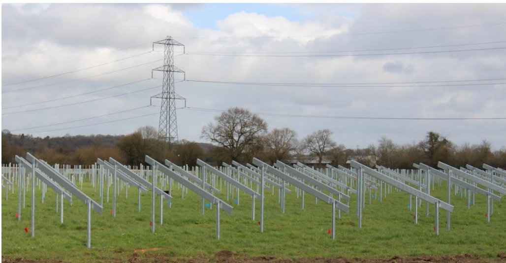
Plate 11c: Installation of Mounting Structures (3 of 4)
