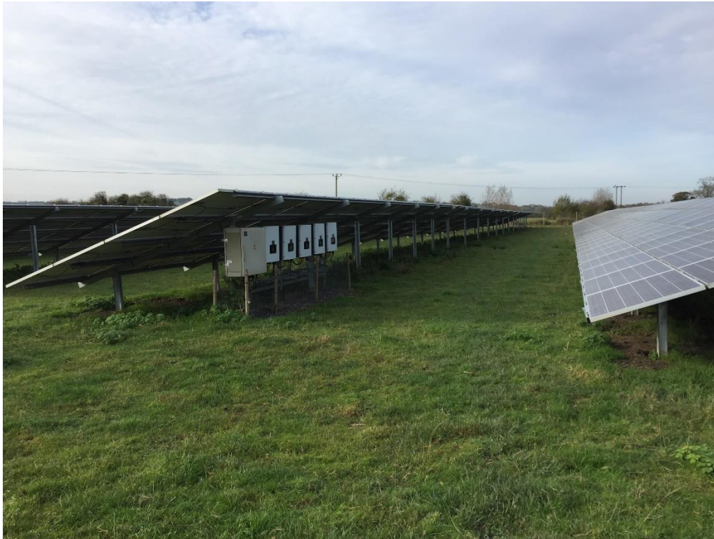
Plate 2 – Example image of string inverters mounted to Mounting Structures beneath the PV Modules
