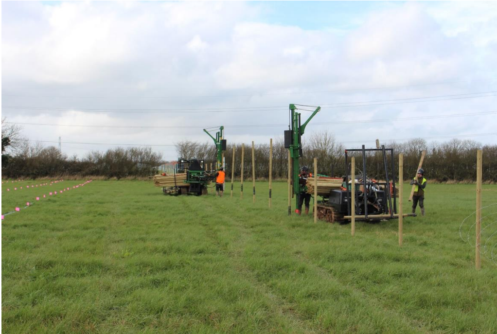
Plate 8: Establishment of Site fencing
