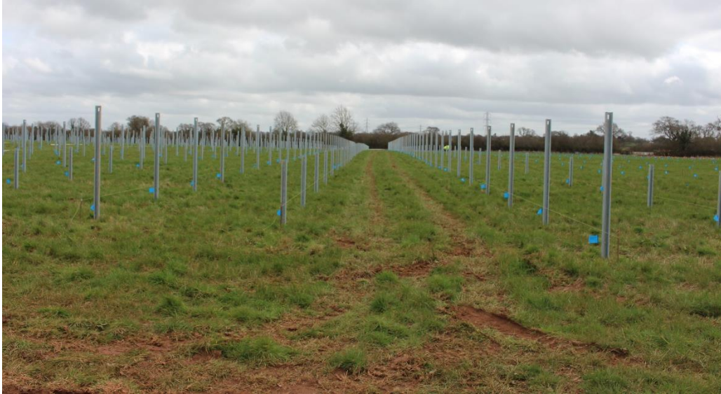
Plate 11b: Installation of Mounting Structures (2 of 4)
